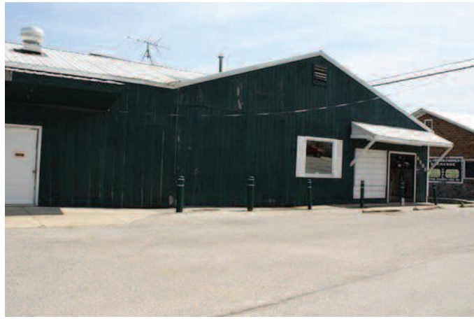
6508 CENTER STREET • ELLSWORTH
